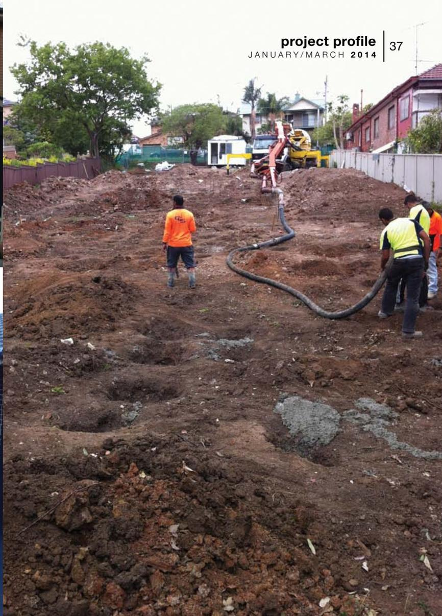
The project involved drilling over 300 piers and almost 80 cubic metres of concrete for the piers and footings. “We had to step every ground floor slab due to the change in levels for every townhouse. Site preparation and all the civil works took time and care”, says Emil.
